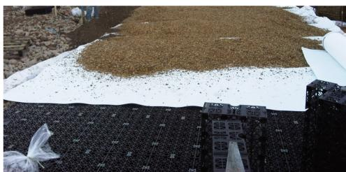
The Permavoid system comprises of high strength modular cells suitable for sub-base replacement, plus components that incorporate silt / oil treatment and shallow flow controls into the system.
