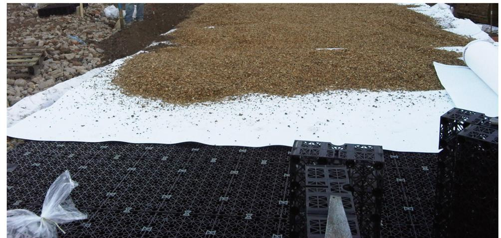
The Permavoid system comprises of high strength modular cells suitable for sub-base replacement, plus components that incorporate silt / oil treatment and shallow flow controls into the system.
