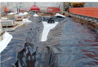
Membrane selection is critical. It needs to be flexible and very robust to deal with the challenges of a brownfield site. Image shows liner to raingarden and position of flow control chamber at the far end, with close up to the left.
